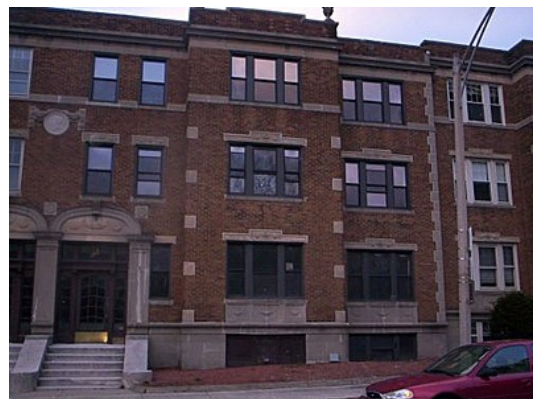
2021 Commonwealth Avenue, Brookline
