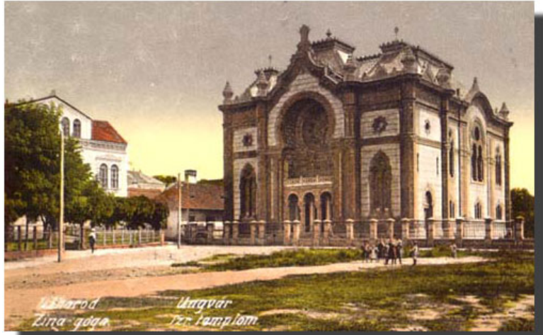
Orthodox Synagogue when built in 1904 with Rabbinate building visible on the left side.
