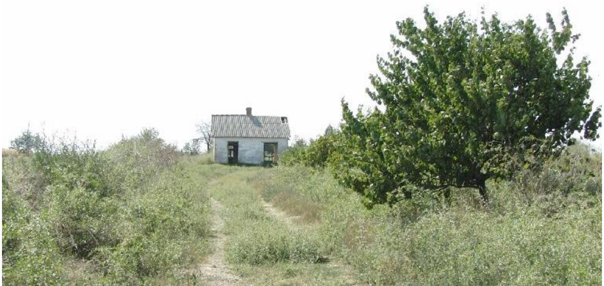
The Cemetery only building in complete abandon seen from the entrance.
